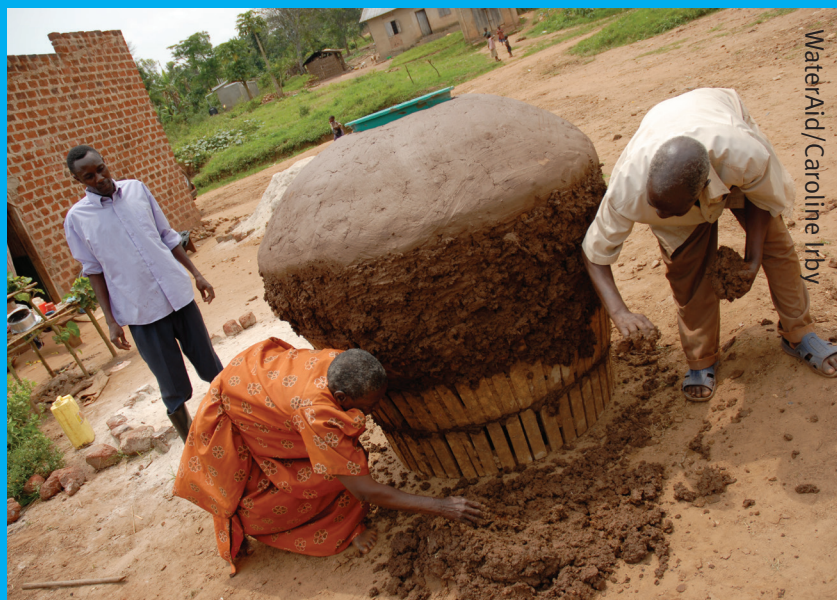
Anna Maria Nanvubya and husband Zevilio Nakuzabasajja Kwafu constructing a rainwater harvesting jar at their home in Kitayita village, Uganda.
